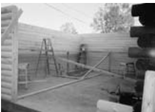
Early construction on the new room addition to HHI's HQ.
